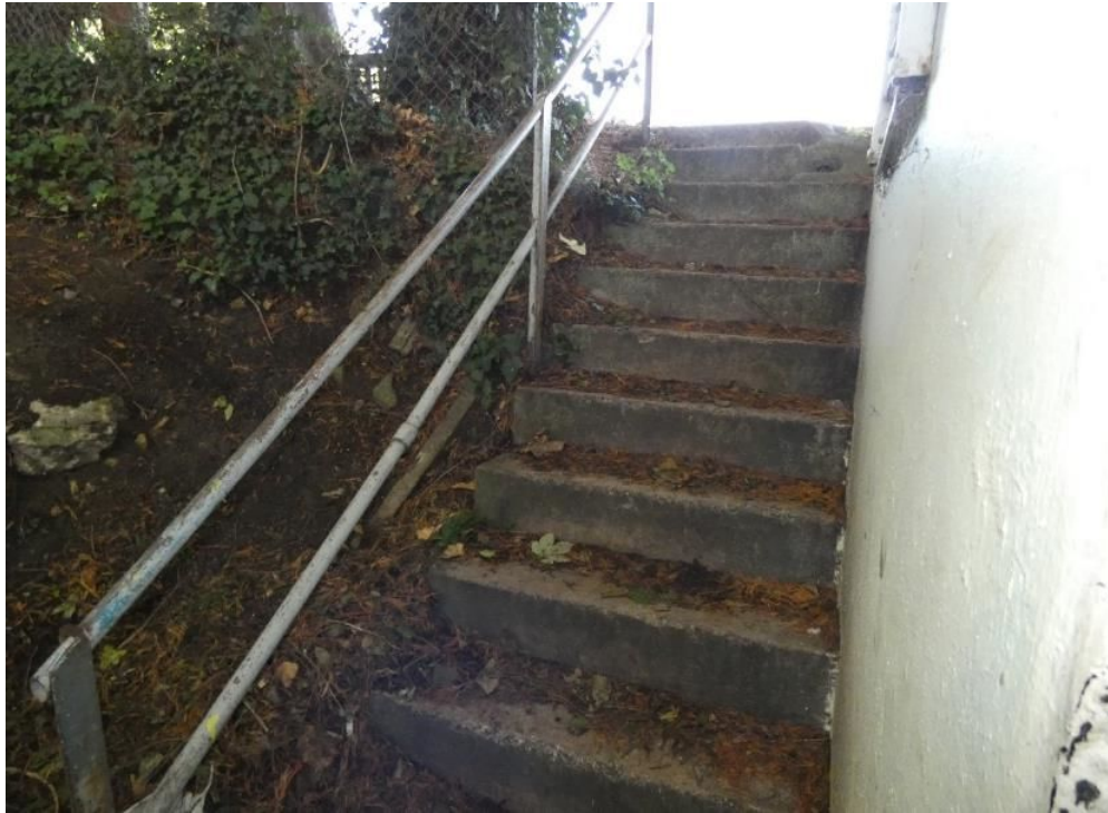
Photograph 13: External steps to the right-hand side.
