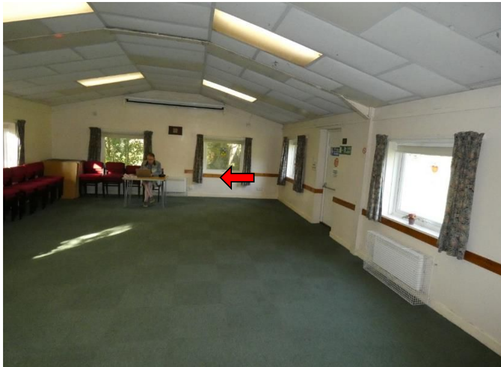
Photograph 8: Factory lining system to the roof of the hall.
