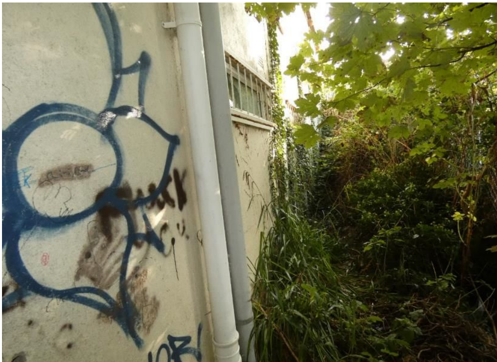
Photograph 2: Inaccessible rear elevation.
