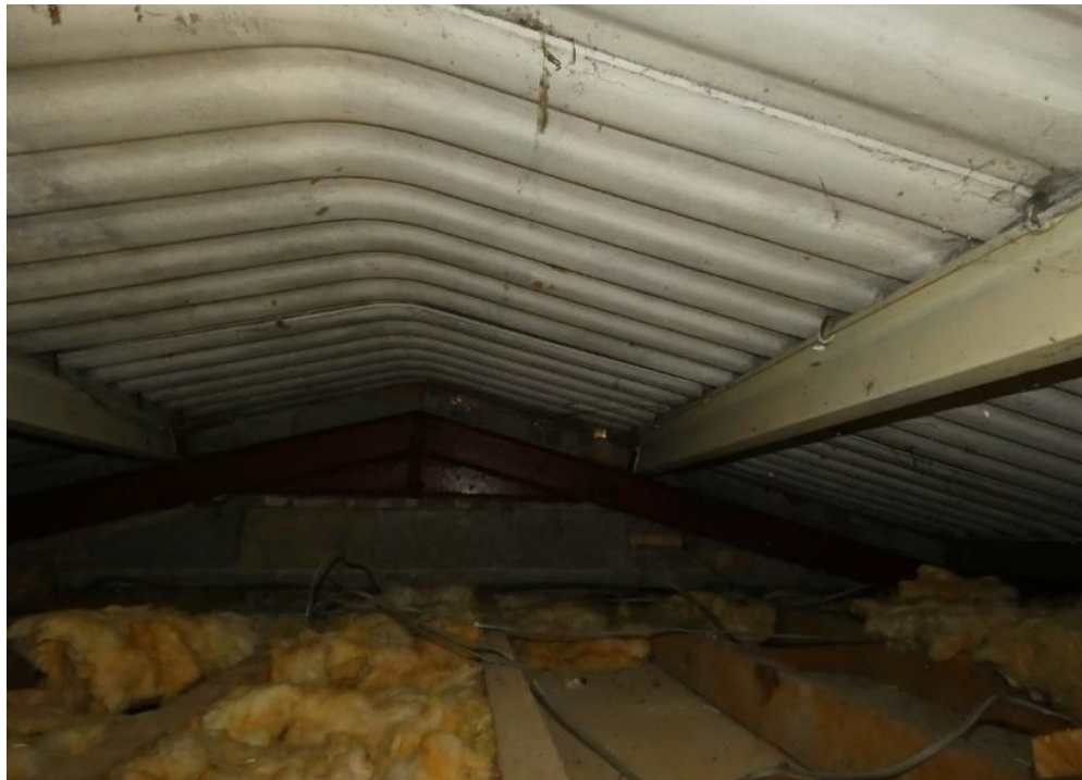
Photograph 6: Roof void over the kitchen.
